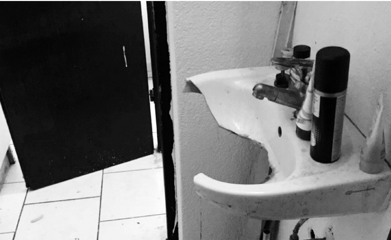
Fig. wet room at Neufrankengasse 6 in October 2015 (Source: Watson, 20.10.2015)
