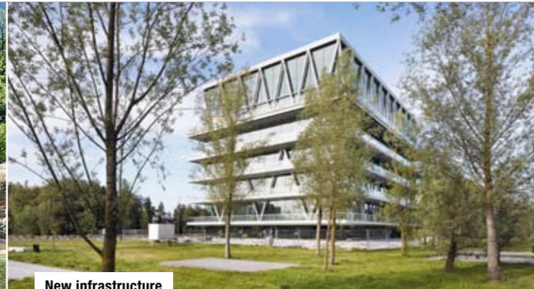
New infrastructure The city is building the Leutschenbach school in the new residential area in the north of Zurich.
