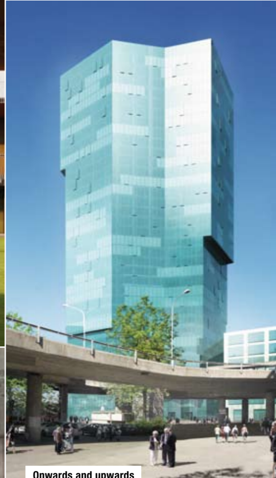
Onwards and upwards New multi-storey buildings are going up in Zurich West, including the new 126 metre-high Prime Tower.
