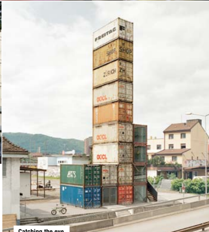
Catching the eye The Gebrüder Freitag Company has its world famous shoulder-bags on sale in a spectacular shop constructed from freight containers.
