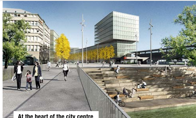
At the heart of the city centre Around the main railway station, a new residential, education and services area is being built – the HB city area.
